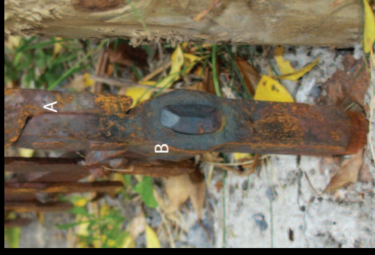
Preparation of a mortice & tenon joint.
