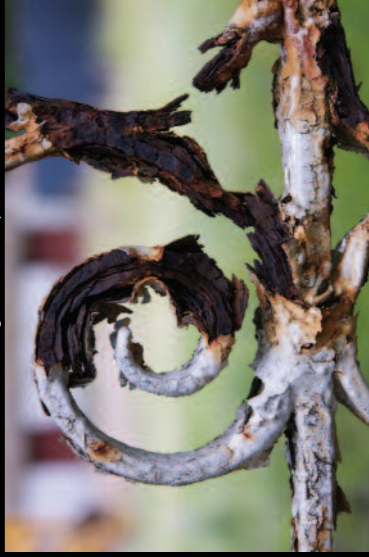
High level of corrosion requiring professional attention.
