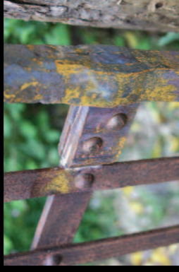
Riveted repair to a traditional gate
