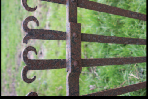
Riveted repair to a traditional gate
