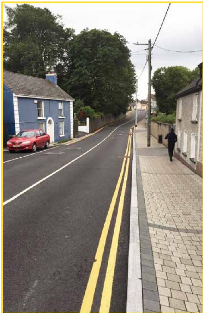
Greensbridge Street completed works
