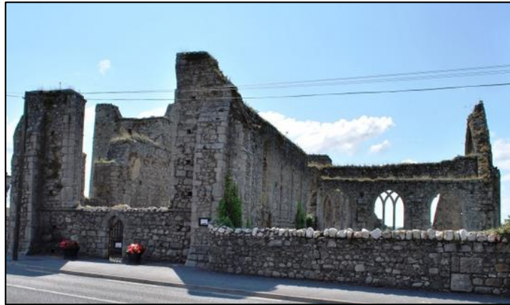
Plate 87 Franciscan Friary at Castledermot, showing transept, through excavation it is known that St Francis' Abbey Kilkenny has a similar layout and it is possible to visualise what the transept would have looked like from this photograph 7 .
