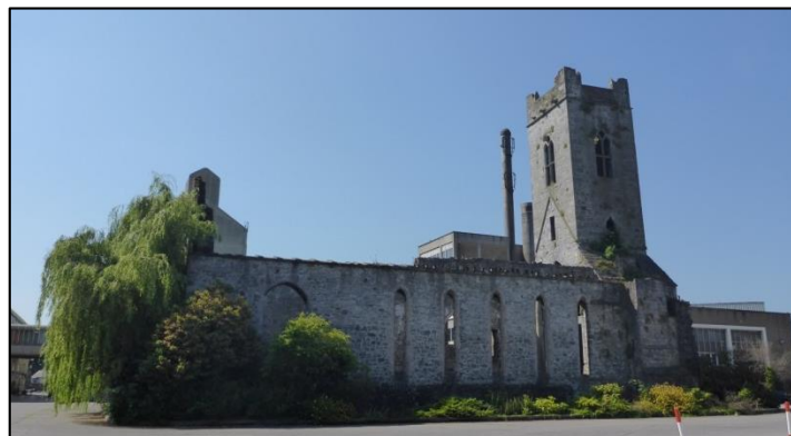
Plate 86 View of St Francis' Abbey taken from the north showing the chancel/choir to the east and tower to the west
