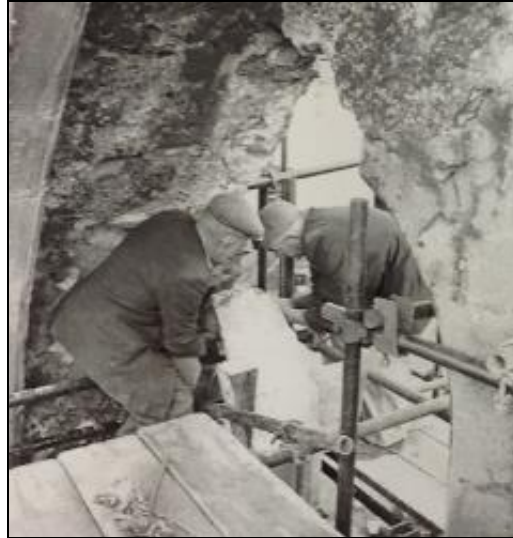
Plate 8 Stone masons at work St Francis' Abbey
