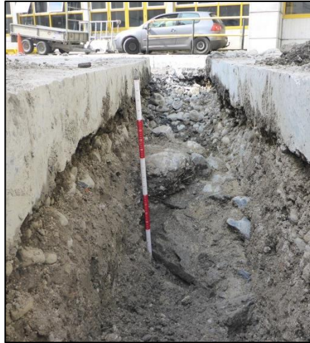
Plate 29 Monitoring ESB trench, culvert section 1
