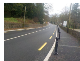
New pavement/footpaths at Discovery Park, Castlecomer.
