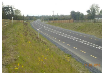
Post Works. View of new Brownstown Junction.
