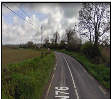
Pre-Works. View North of Brownstown Junction
