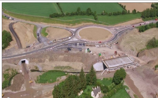
Construction Works at Glenmore Roundabout and road underpass
