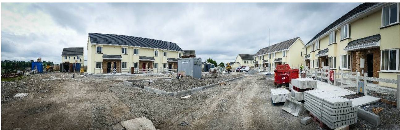
Housing at Togher Way under construction
