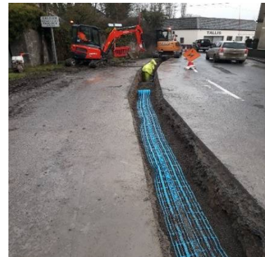
Installation of new watermain by Directional Drilling in Freshford
