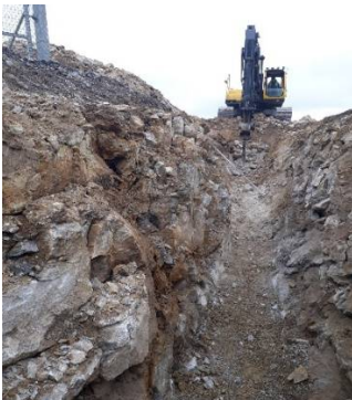
Installation of Back wash pipe from Galmoy WTP
