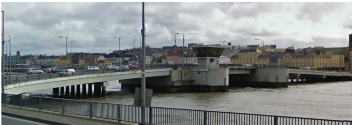
Rice Bridge Over River Suir
