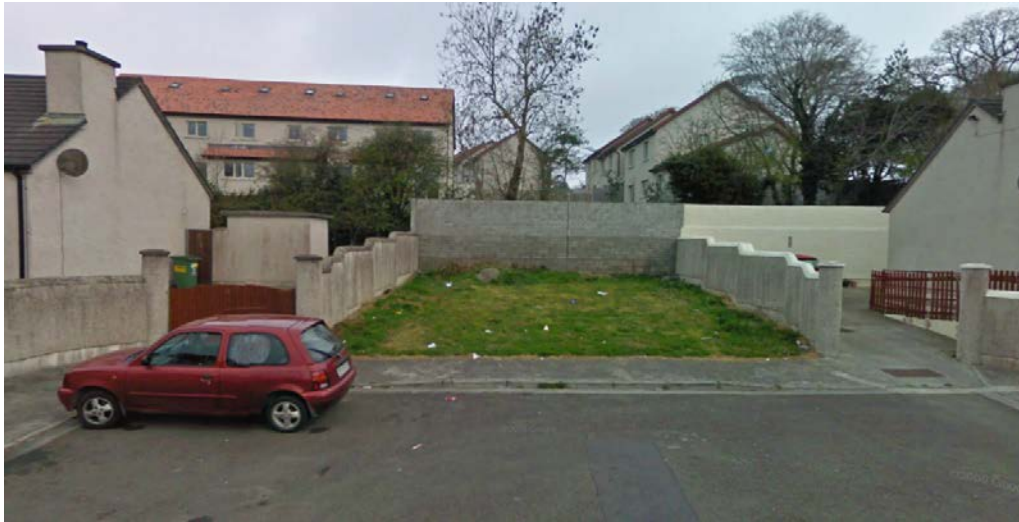
Photo: Árd Doire - Wall between Oak Ridge and Árd Doire
