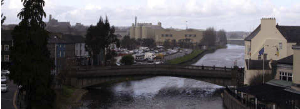
Plate 11.2 View of the proposed River Nore bridge crossing looking north from the high grounds of Kilkenny Castle
