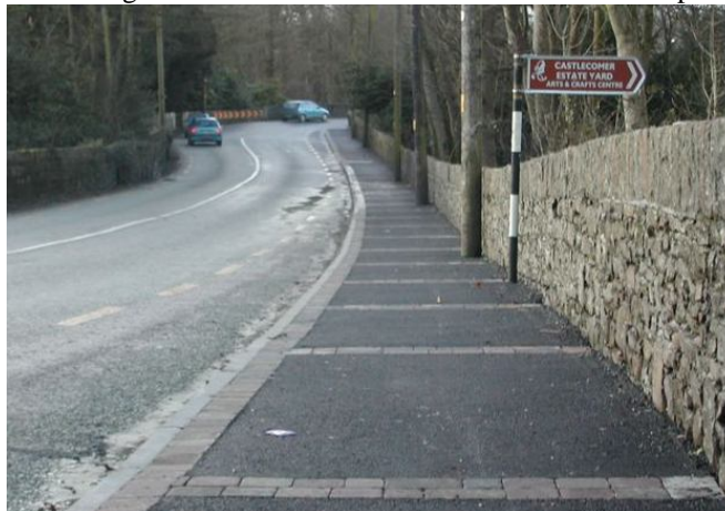
New footpath at Athy Road, Castlecomer
