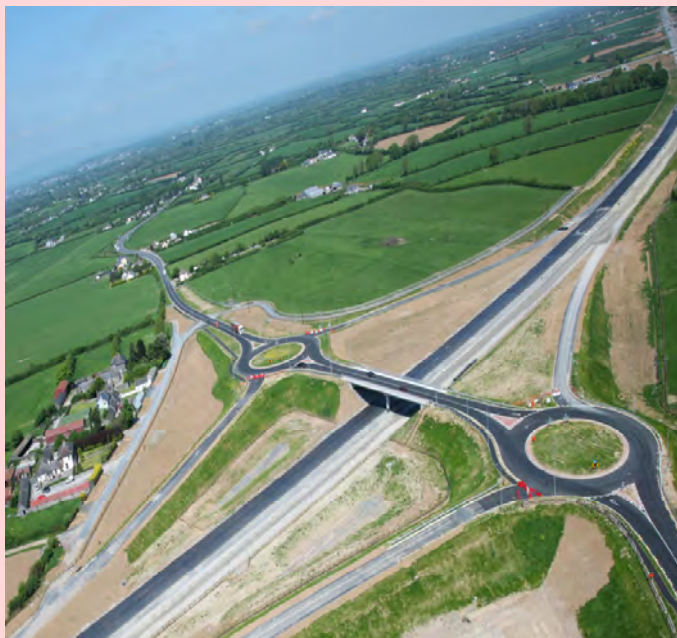
Realigned N62 at the Horse & Jockey Interchange
