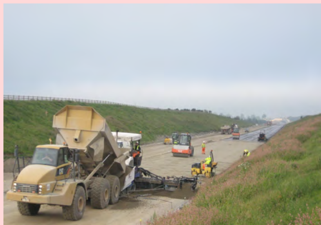
CBM Pavement Works North of Twomileborris
