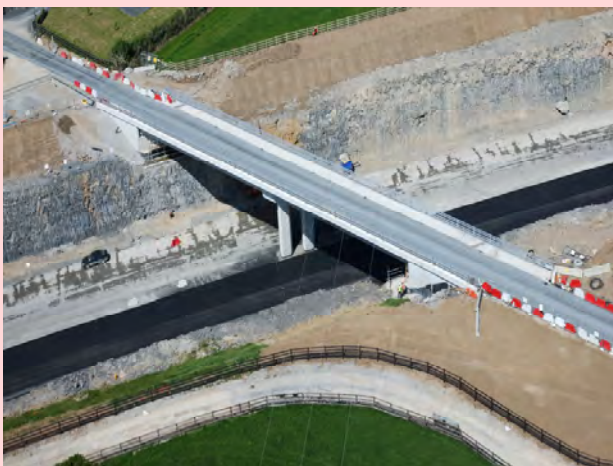
Structure 104 at Grangemore Cashel
