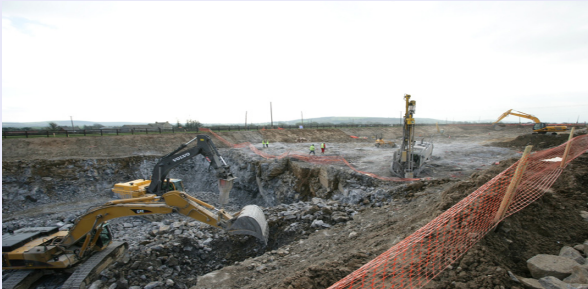
Rock Excavation at Grangemore, Cashel
