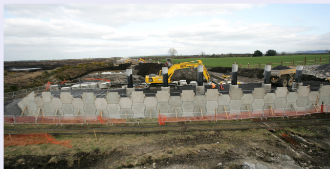
Abutment to Structure 120 Bord Na Mona Railway Bridge
