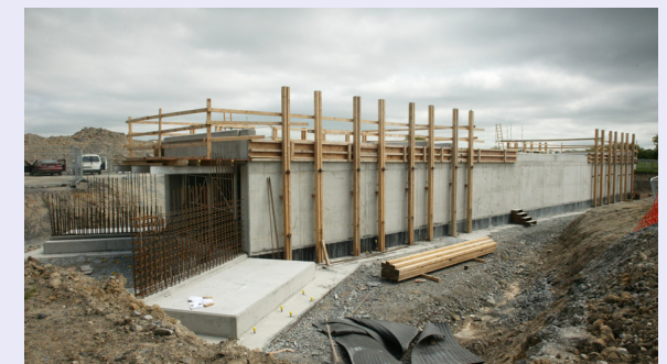
Farm Underpass at Two Mile Borris
