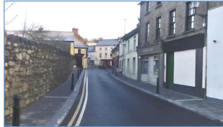
Pipe Street – After
