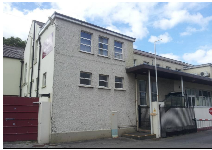
3. View of raised walkway and Canopy from South west
