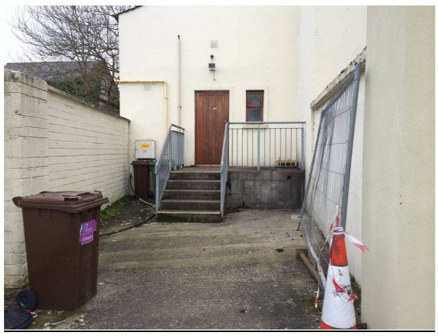
2. View of Service Yard adjoining West façade
