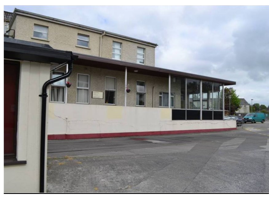
4. View from Horse Barrack Lane (South)
