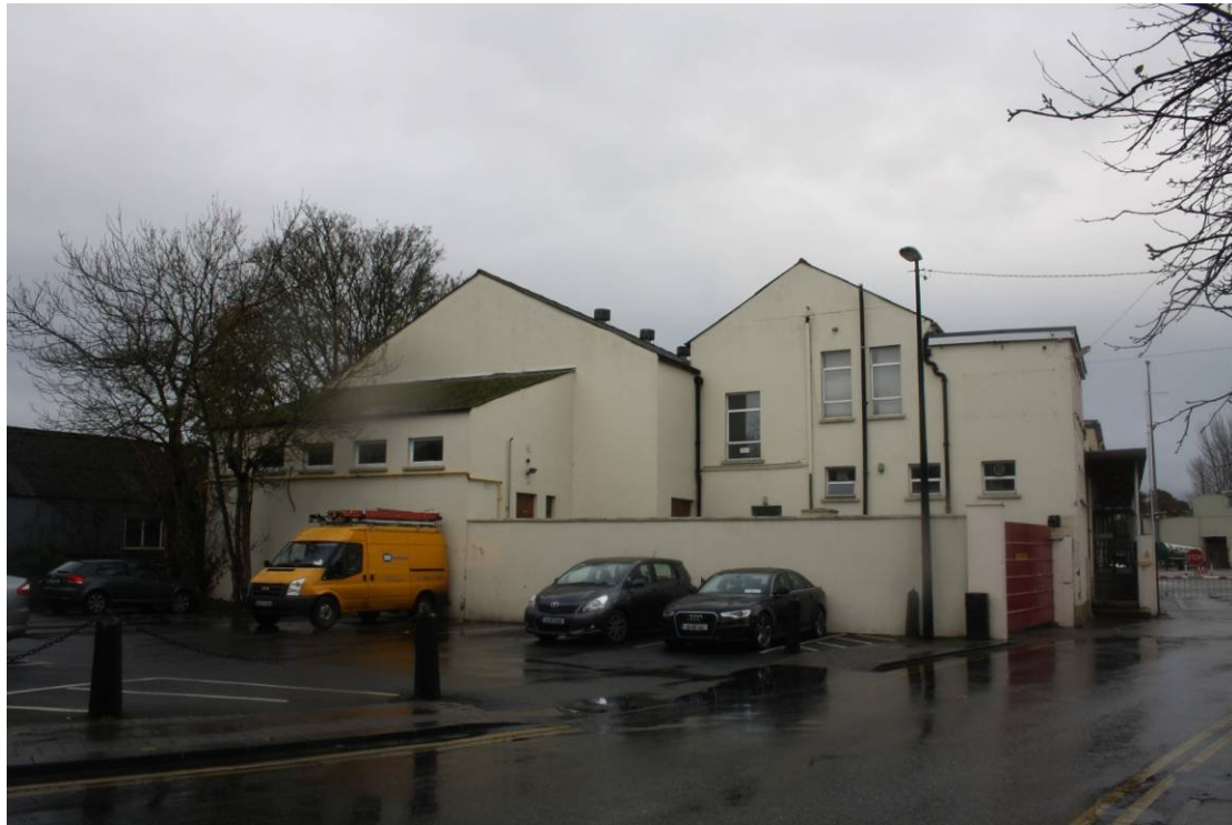
Figure 18: The Mayfair building, from the southwest
