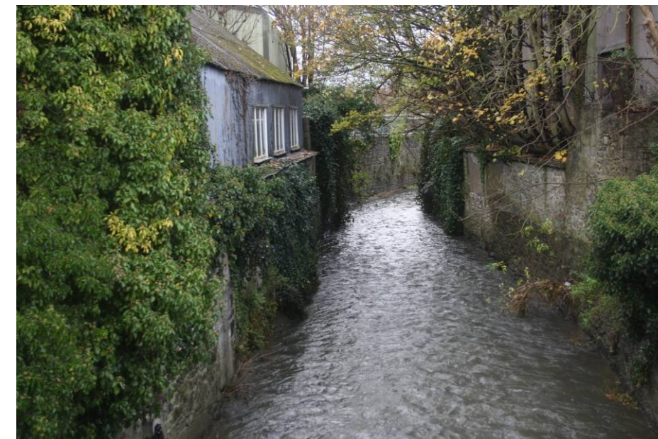
Figure 8: The Town Wall from Watergate Bridge
