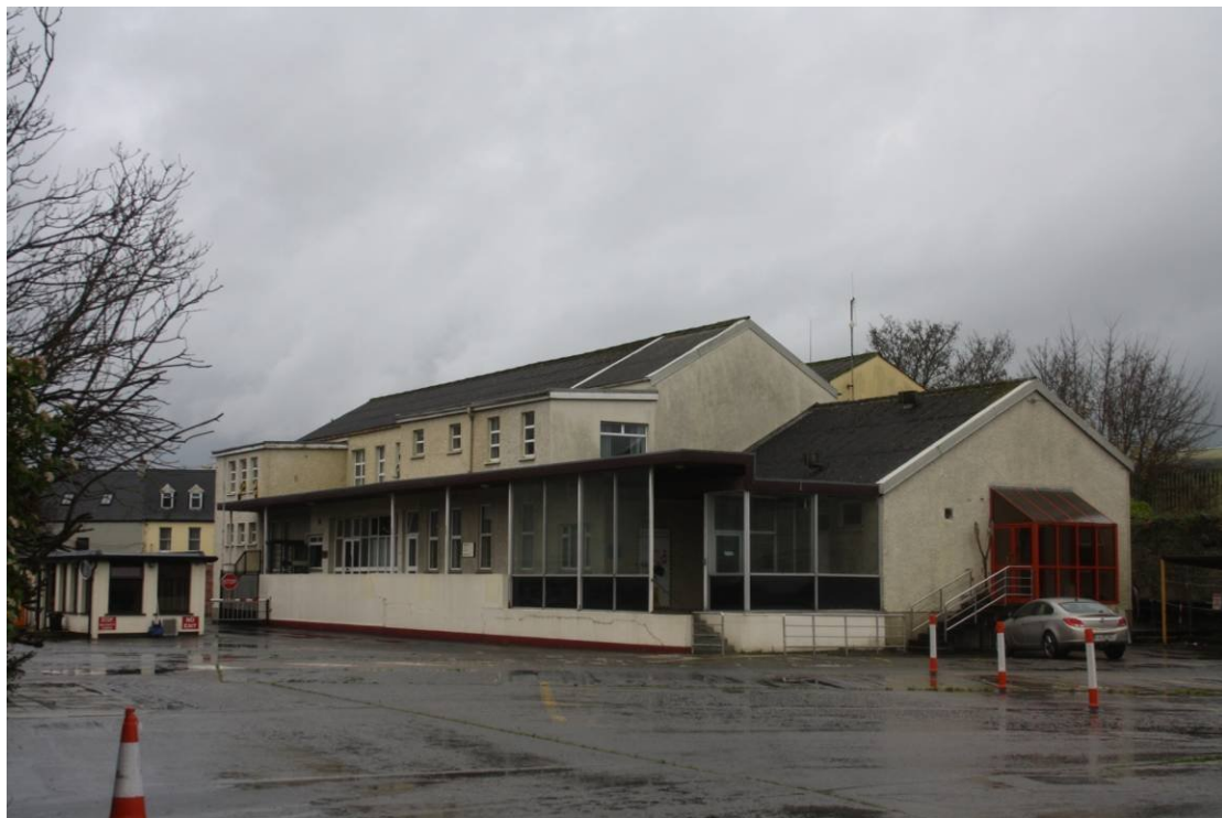
Figure 19: The Mayfair building, from the southeast
