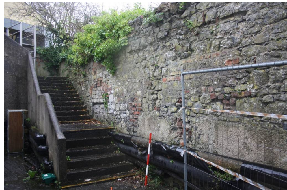
Figure 23: Blocked arrow loops in Town Wall adjoining Mayfair building
