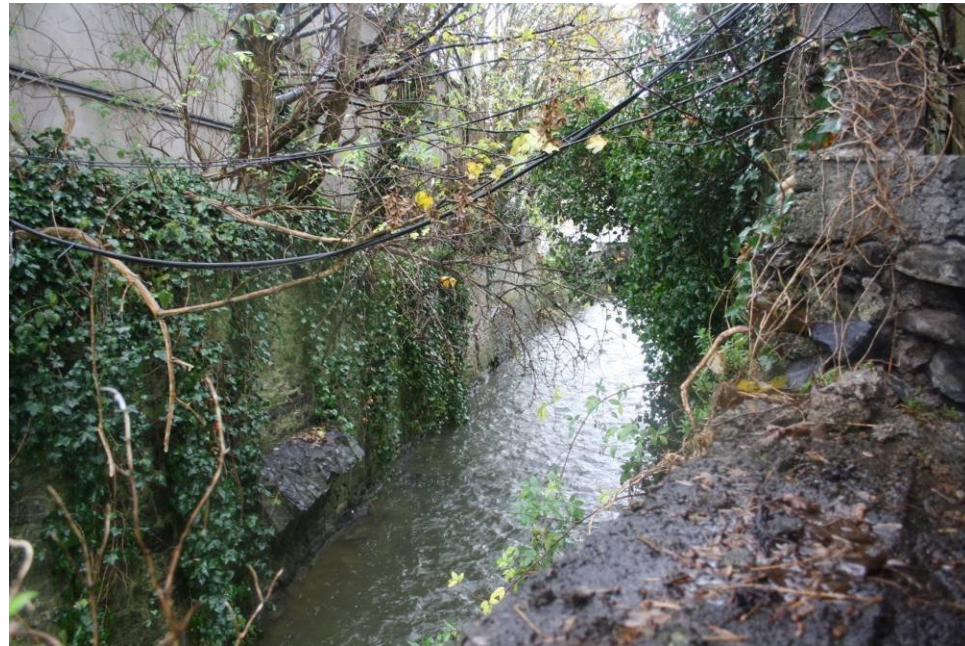
Figure 22: Truncated arch in the Town Wall, from northeast
