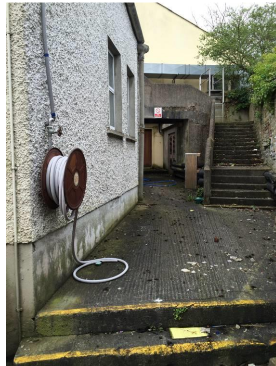
View of concrete steps along city wall
