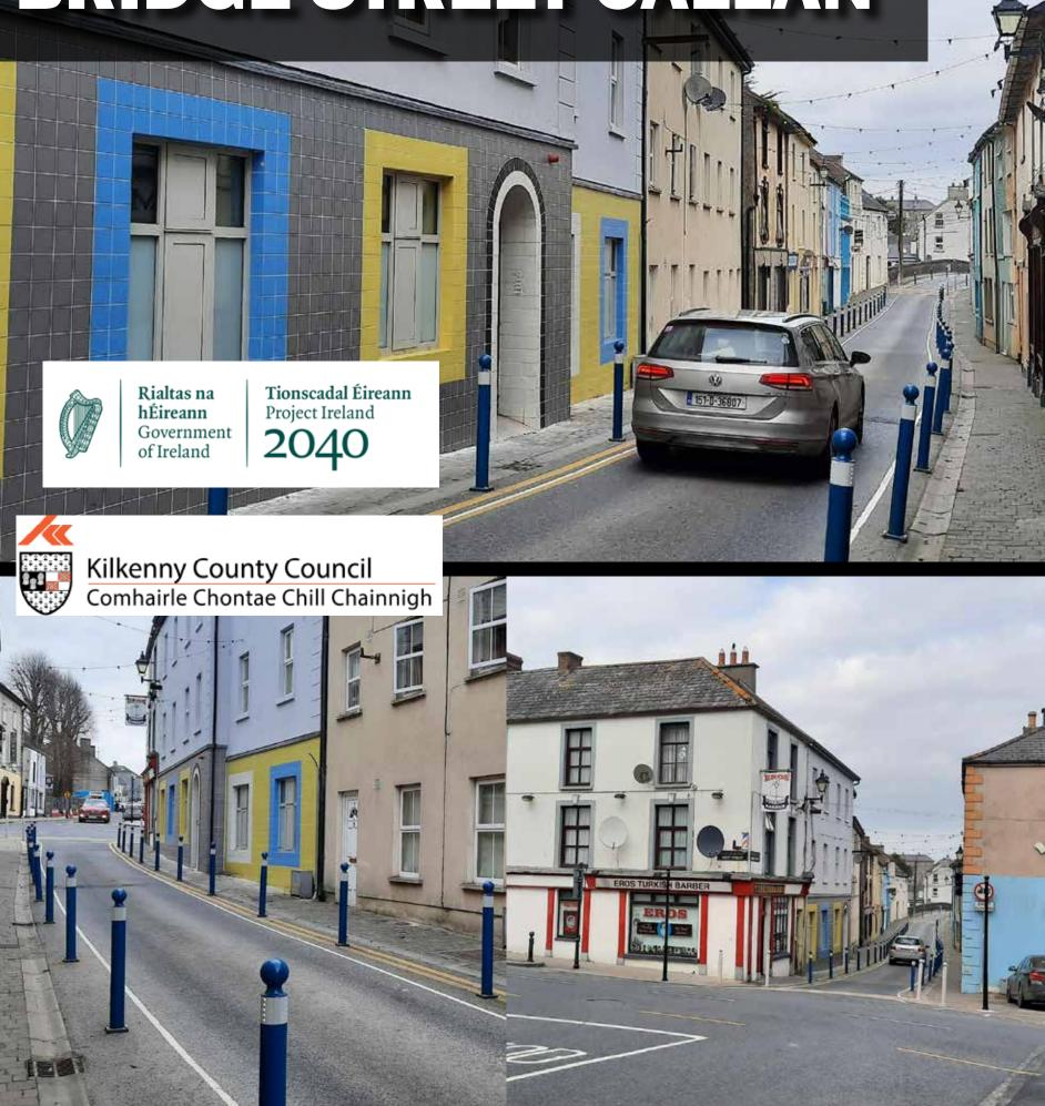
Funding was secured by Kilkenny County Council towards the improvement of the public realm space on Bridge Street and to accommodate shared surfaces for walking whilst improving social distancing. Bollards, road markings, signage and realignment works at the junction were carried out.
