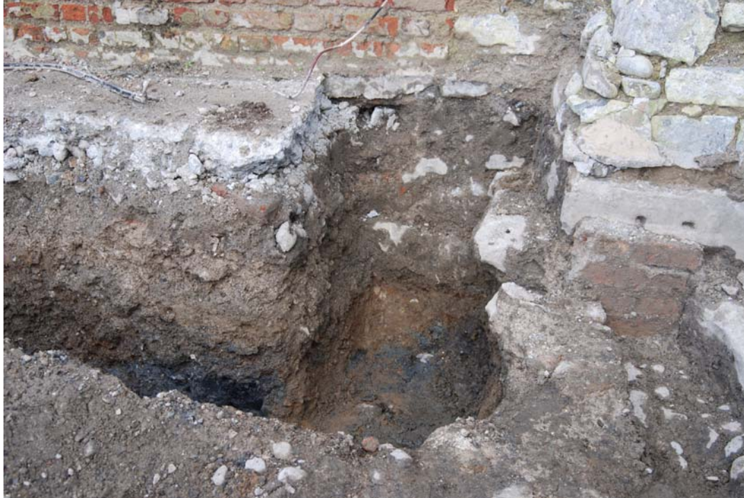
Plate 10: Test Trench 4 showing foundations of west front long wall of No 22 Vicar St, and underlying cobbles (C015) (centre of pic), and bricked up drain (C021) and cobbles (C012) at base, and re-used chamfered stone (right of pic), facing east.
