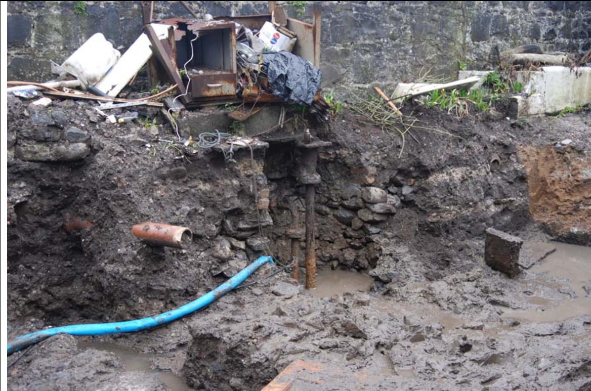
Plate 17: Test Trenches 7 & 8 showing modern water pump and cut (C128), facing north
