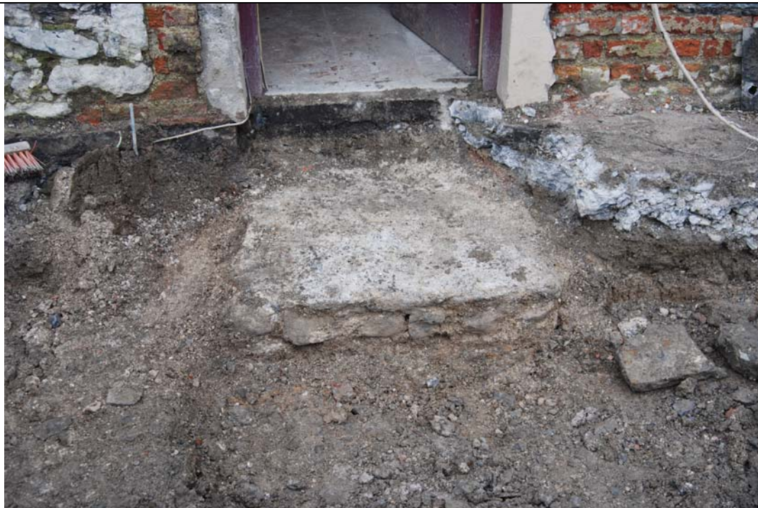
Plate 9: Test Trench 4 showing compacted mortar layer (C165) and cobbles (C172) forming old doorway in No 22 Vicar St, facing east.
