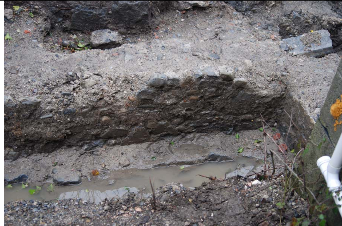
Plate 23: Test Trench 9 showing wall (C060) and footings, facing north. This wall is shown on Rocque's Map (1758) and 1 st ed OS map (see Fig 14). It is proposed to remove this wall and establish if any archaeology remains below at this location.
