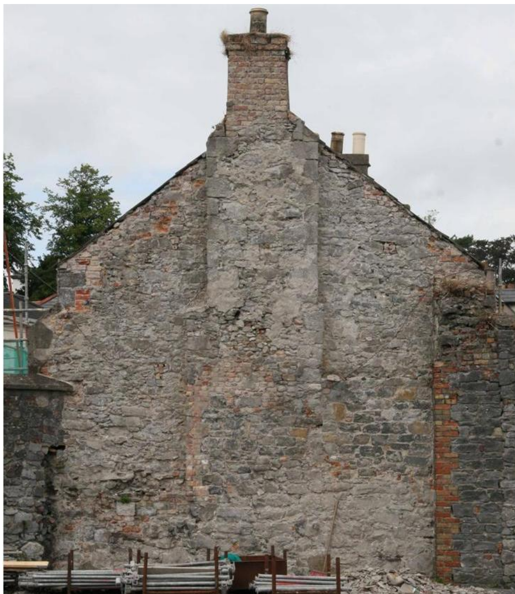
Plate 13: Southern face of gable wall
