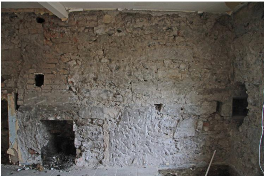
Plate 10: Interior of gable wall at ground floor - right
