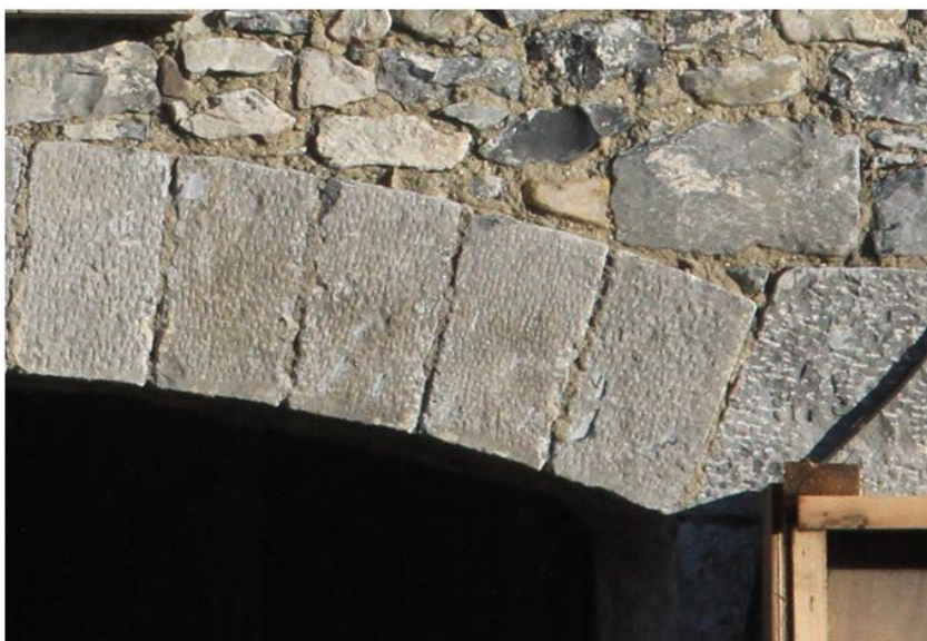
Plate 6: Cut stone in the arch over the carriageway
