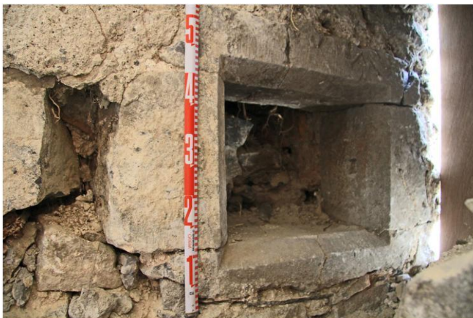
Plate 8: Stone-lined opening in gable wall
