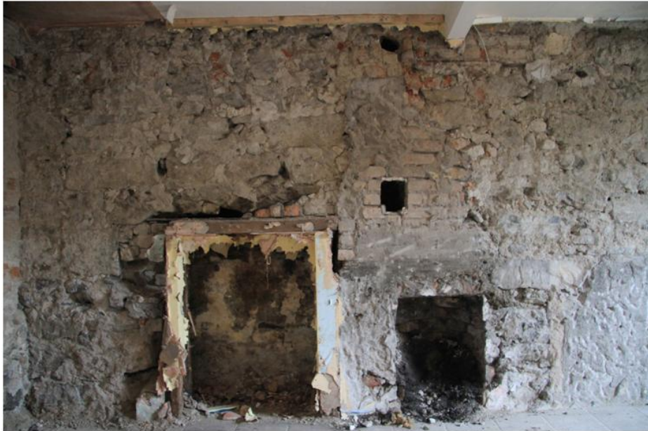
Plate 9: Interior of gable wall at ground floor - left
