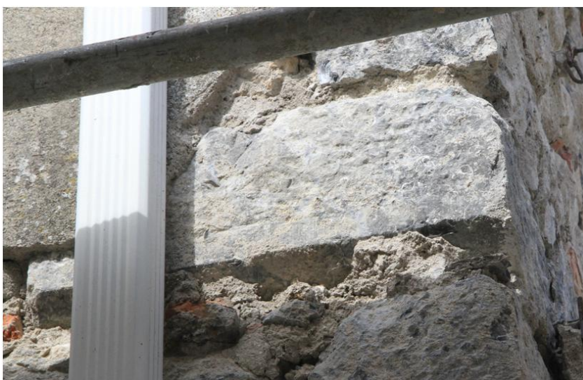
Plate 5: Chamfered stone window or door jamb in return at rear
