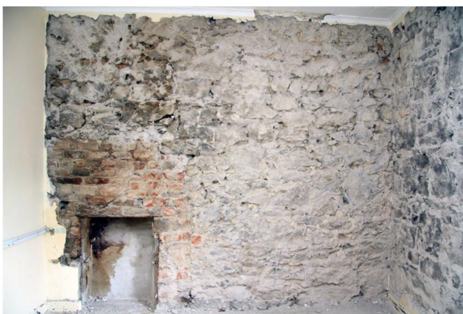
Plate 12: Gable wall, seen in larger first floor room
