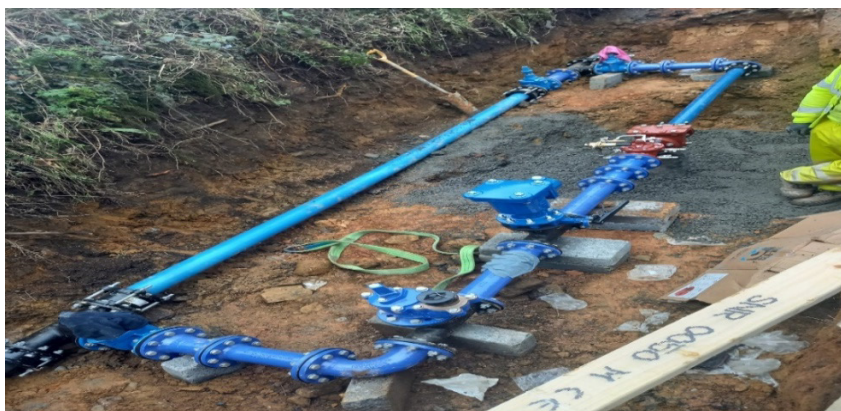
PRV installation at Kiltown Cross, Inistioge
