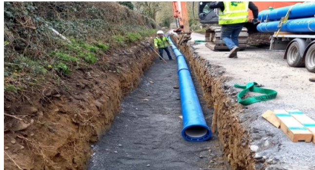
Construction of Ductile Iron Rising Main to Rathduff Reservoir
