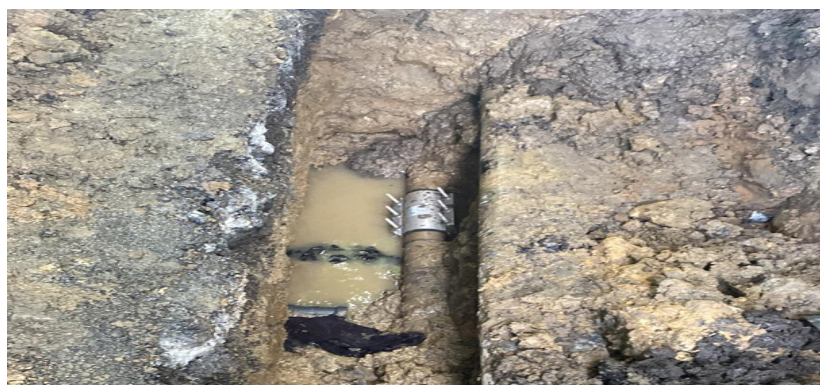
Find and Fix Leak repair at Kilcross, Inistioge
