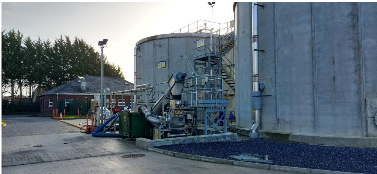
Kilkenny City & Environs Wastewater Treatment Plant Purcellsinch Completed Sludge Import Screen & Wash Press
