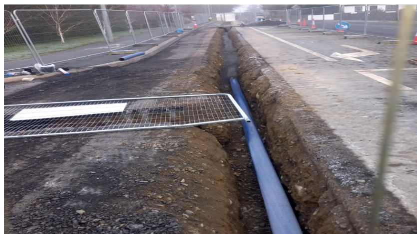
Construction of new HDPE watermain at Dublin Rd, Thomastown
