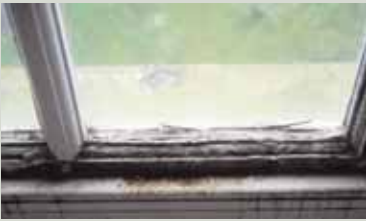
This mid eighteenth-century oak sash was dipped before being repaired with new parts. The ultimate effect of the chemical on the oak is obvious and serious: the original fabric is now incapable of repair
