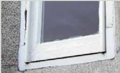
The new ends on these recently repaired stiles were not cut at an angle and the paintwork is starting to flake. Both factors will make the new joints prone to moisture ingress, which could start to damage the joint and soften the timber
