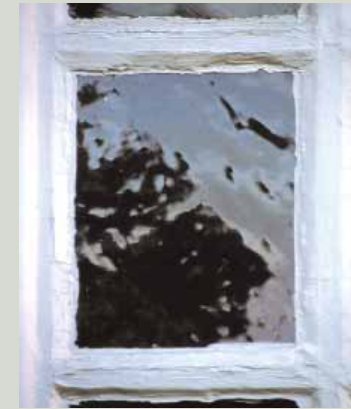
Early cylinder glass has an extremely hammered looking surface and is quite speckled with bubbles or seeds, like the pane in this early eighteenth-century window
