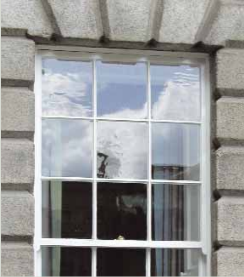
This sash was glazed with modern cylinder sheet glass. Each sheet of this or any other substitute for historic glass should be carefully examined before using it, as some, especially those sold for stained glass work, contain exaggerated imperfections and will look out of place
