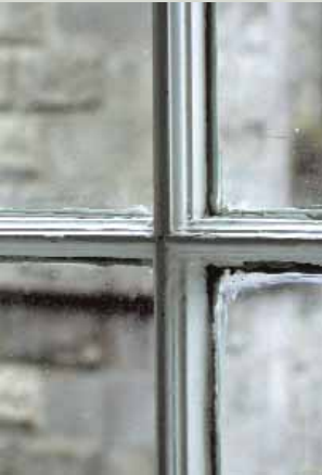
At some stage one of the glazing bars in this sash was repaired (vertical bar, top half of picture). While this kept the sash in use, a standard moulding was used instead of a profile matching the late eighteenth-century original. Small details like this should not be overlooked by those in charge of a repair job
