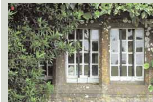
Lead-glazed fixed lights and casement windows of the seventeenth century are extremely rare in Ireland. Called 'quarry glazing', lead panels were still being made into the early eighteenth century, but were seen as inferior to timber-framed windows in every way
