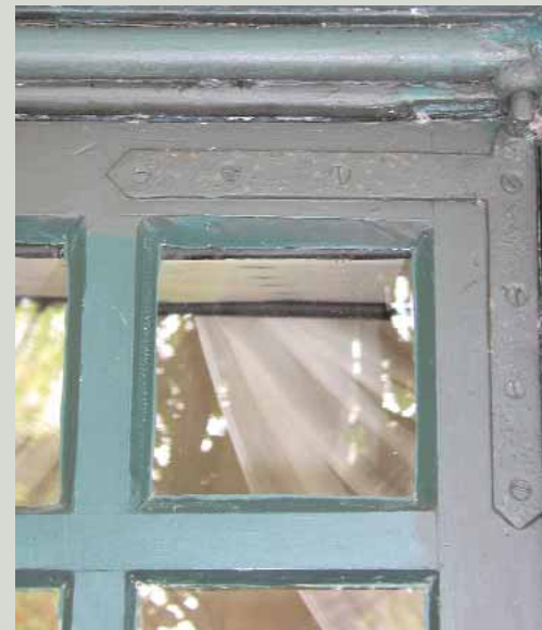
Wrought iron is generally resistant to corrosion and is capable of repeated repair unless it has worn very thin. The hinges of this early nineteenth-century window are substantial and should continue to work for many years
