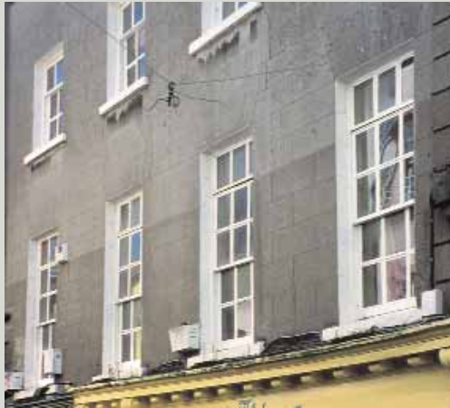
It may be that making a separate top row of panes was a practical answer to reducing the weight of the upper sash. Whatever the reason, it is a feature unique to Wexford and should be appreciated and conserved where it survives
