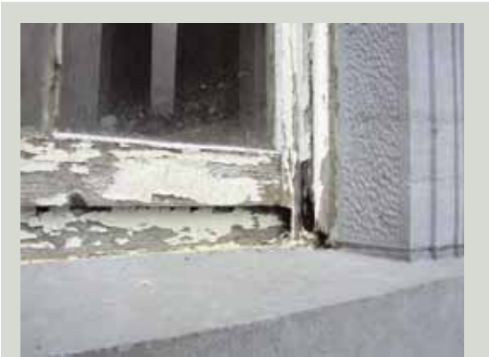
The loss of paint should not be the main guide as to the condition of the timber. Despite years of neglect, this window did not require substantial replacement of timbers. The ends of the box frame and its linings, as the most vulnerable areas, did require new scarfed repairs
