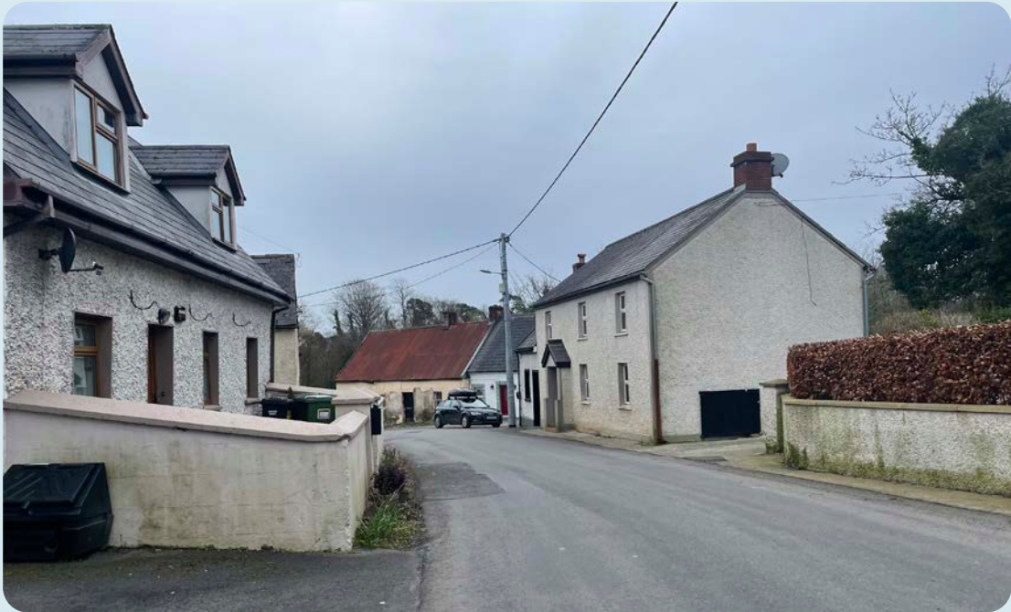
Figure 3.13: Absence of footpaths, Kilmacow lower
