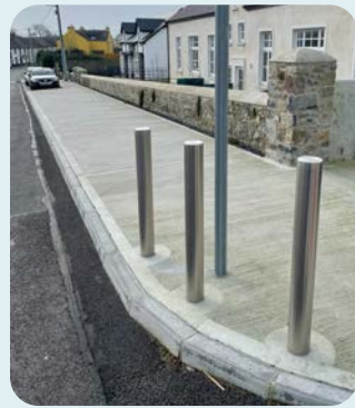
Figure 3.35: Improved footpaths at the Old Creamery
