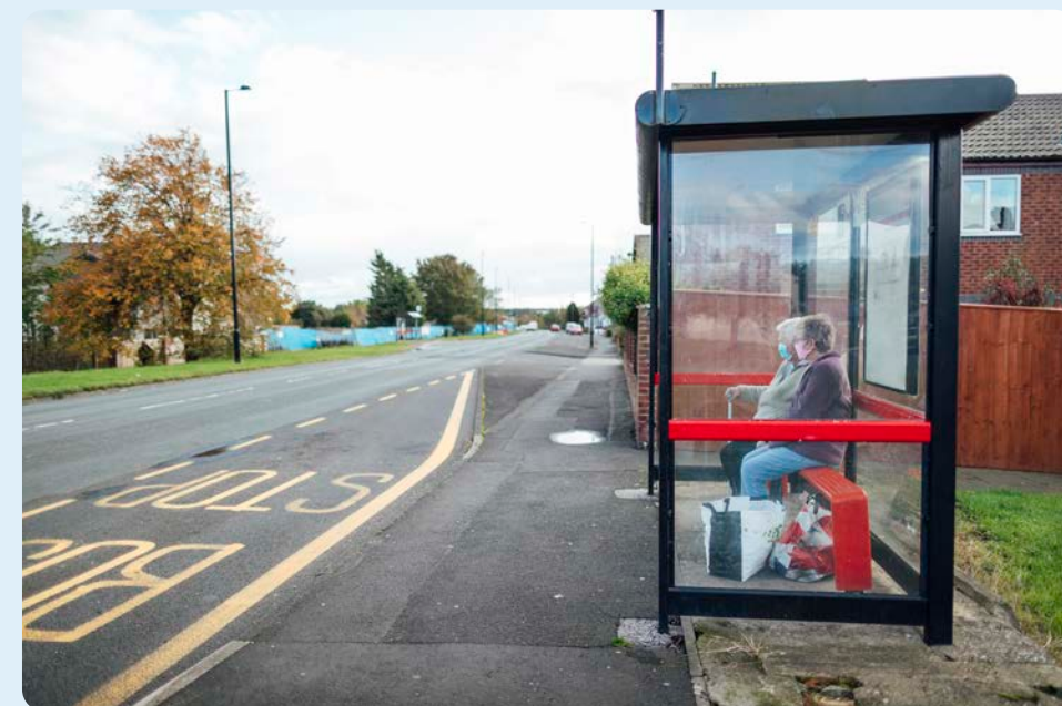
Figure 5.19: Example of bus shelter
