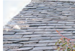
Traditional roof coverings and chimney stacks
