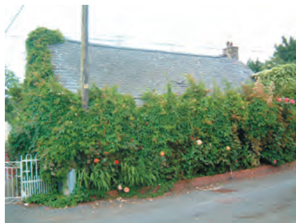
Traditional vernacular single storey cottage with slate roof
