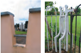
Frontage walls and boundaries
