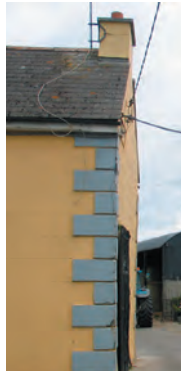
Detail showing quoins along the corner
