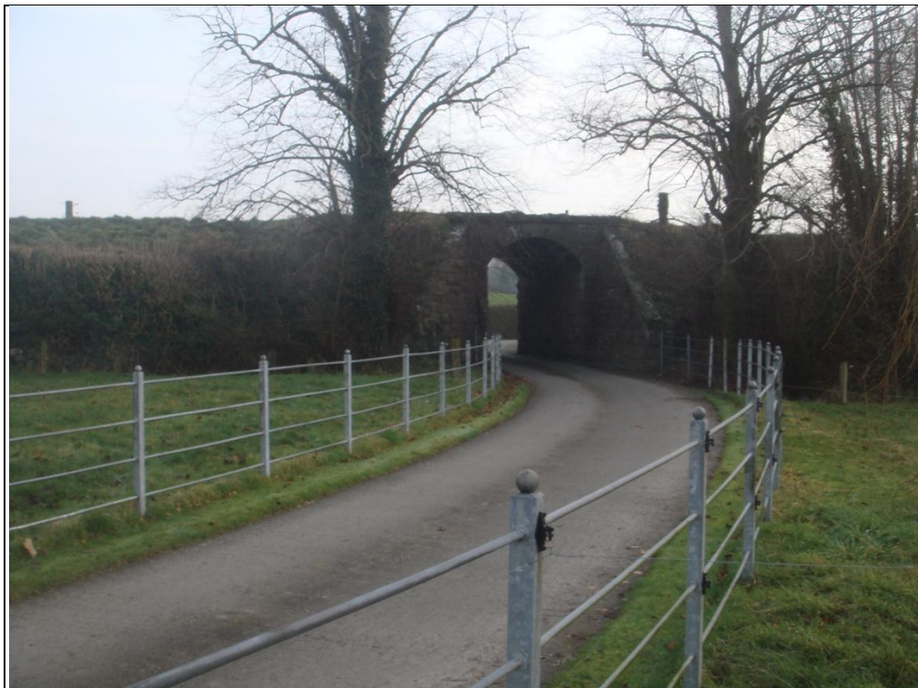
Plate 13.14 View of surviving underpass of former GSWR railway at Dunmore House
