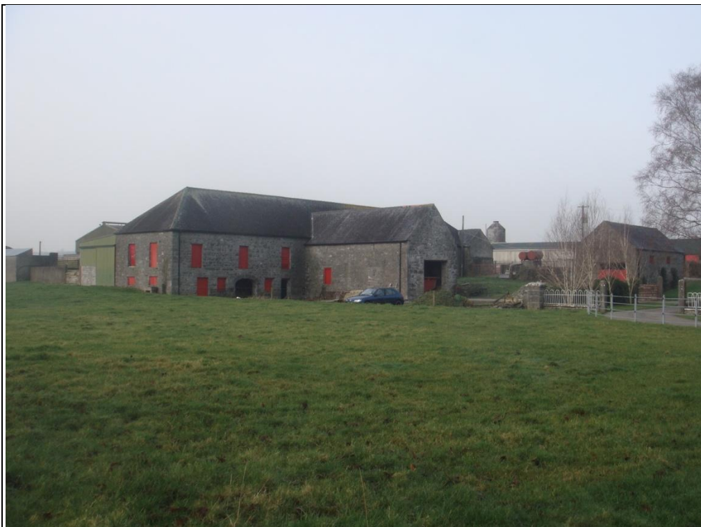
Plate 13.18 Farm complex AH 4 – view of farm buildings from southeast
