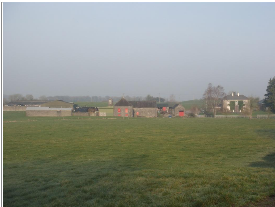
Plate 13.12 Farm complex AH 4 viewed from the proposed route
