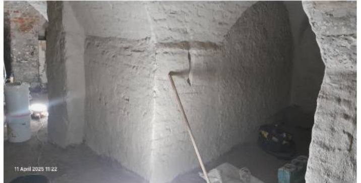
Limewash ongoing in basement
