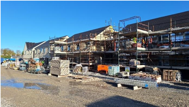
20 houses under construction at An Tobar, Freshford
