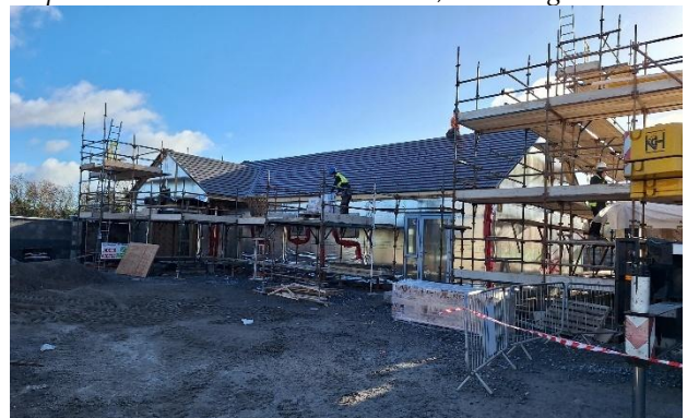
Group home under construction at An Tobar, Freshford
