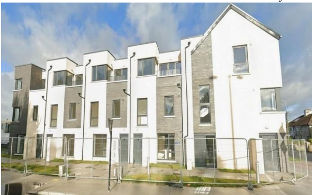
Apartments at Marnellsmeadows, College Road
