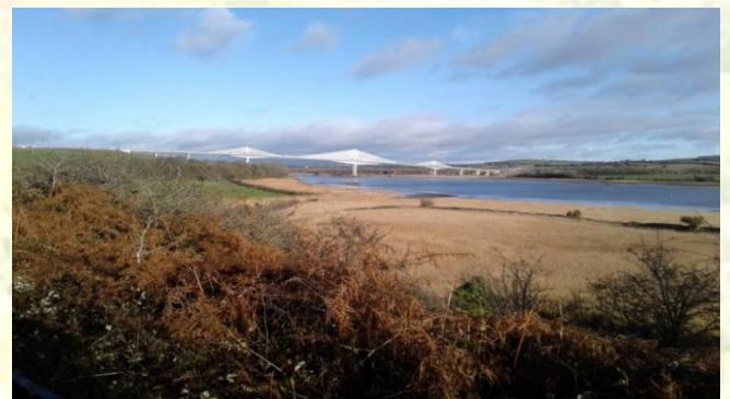
View of the Rose Fitzgerald Kennedy Bridge from the railway line at Carrickcloney
