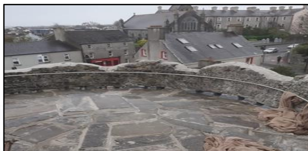
View from the newly repaired roof at Talbot’s Tower
