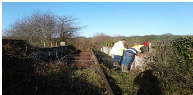
Examining the old bridge structures following vegetation clearance
