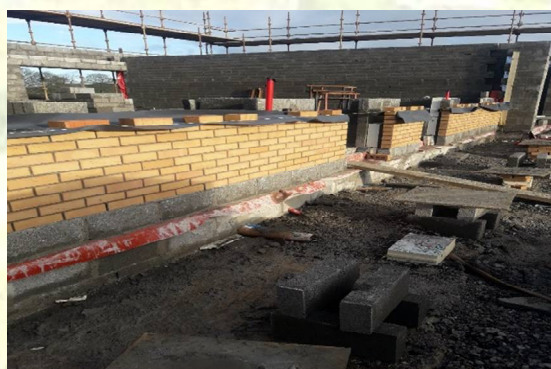
22 houses under construction at Station Road, Ballyraggett
