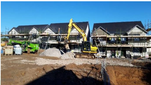
17 units under construction at Breagh Place, on Main Street, Piltown
