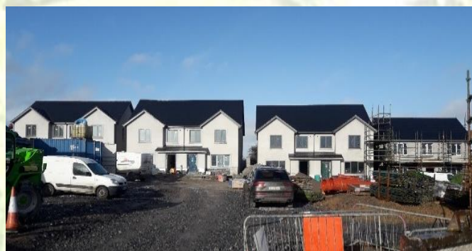
Breaghagh Place, Piltown – 17 units under construction
