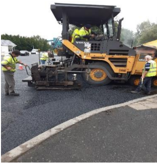
Paving works at Kilkenny Road Callan
