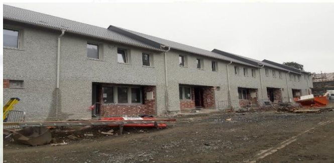
Glebeside, Donaguile, Castlecomer 33 units under construction
