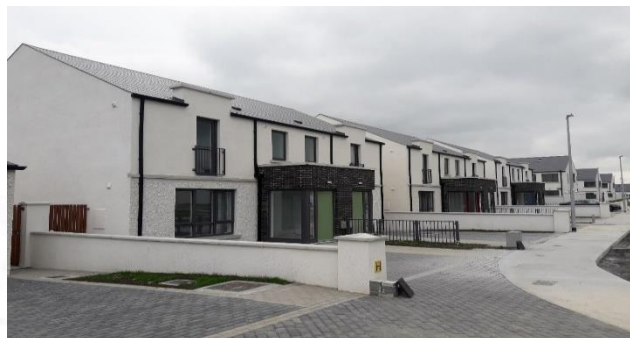
Completed Scheme at Hoban Park, Bolton, Callan
