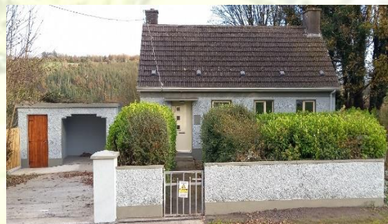
Old Health Centre, Windgap ready for occupation
