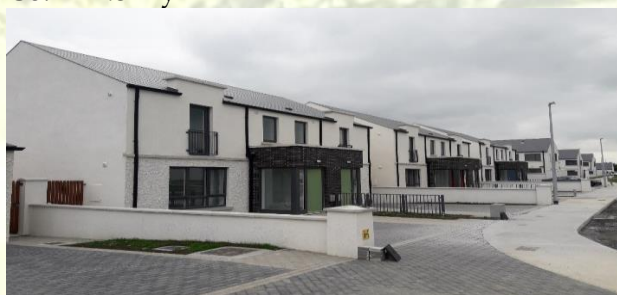
Completed Scheme at Hoban Park, Bolton, Callan
