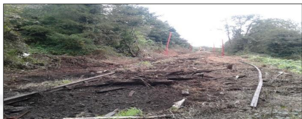
Clearance of rails and sleepers along the line of the old railway track at Rathpatrick, Slieverue
