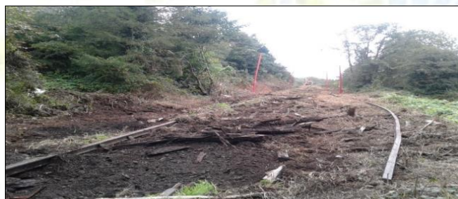
Lifting of old rails and sleepers along the route of the South East Greenway
