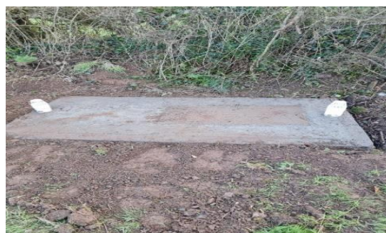
New Cover provided to existing Septic Tank following inspection
