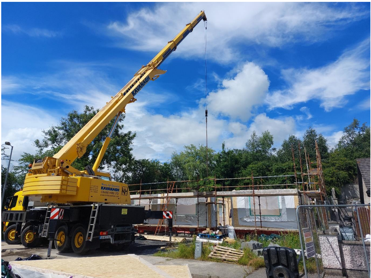
Erection of timber frame at Inchacarron Mullinavat. Low Carbon Construction
