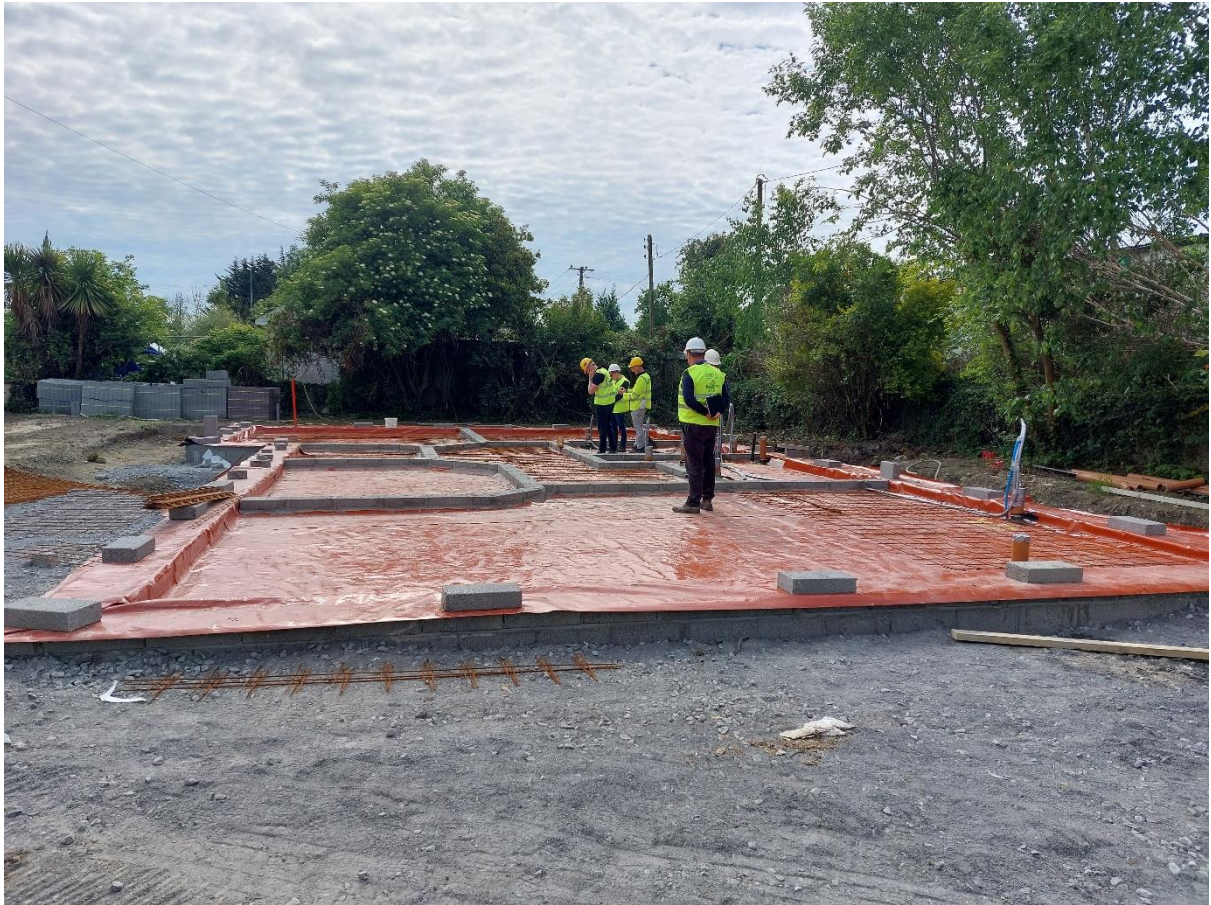
3 bed accessible house at Haggardsgreen, Callan – substructure complete
