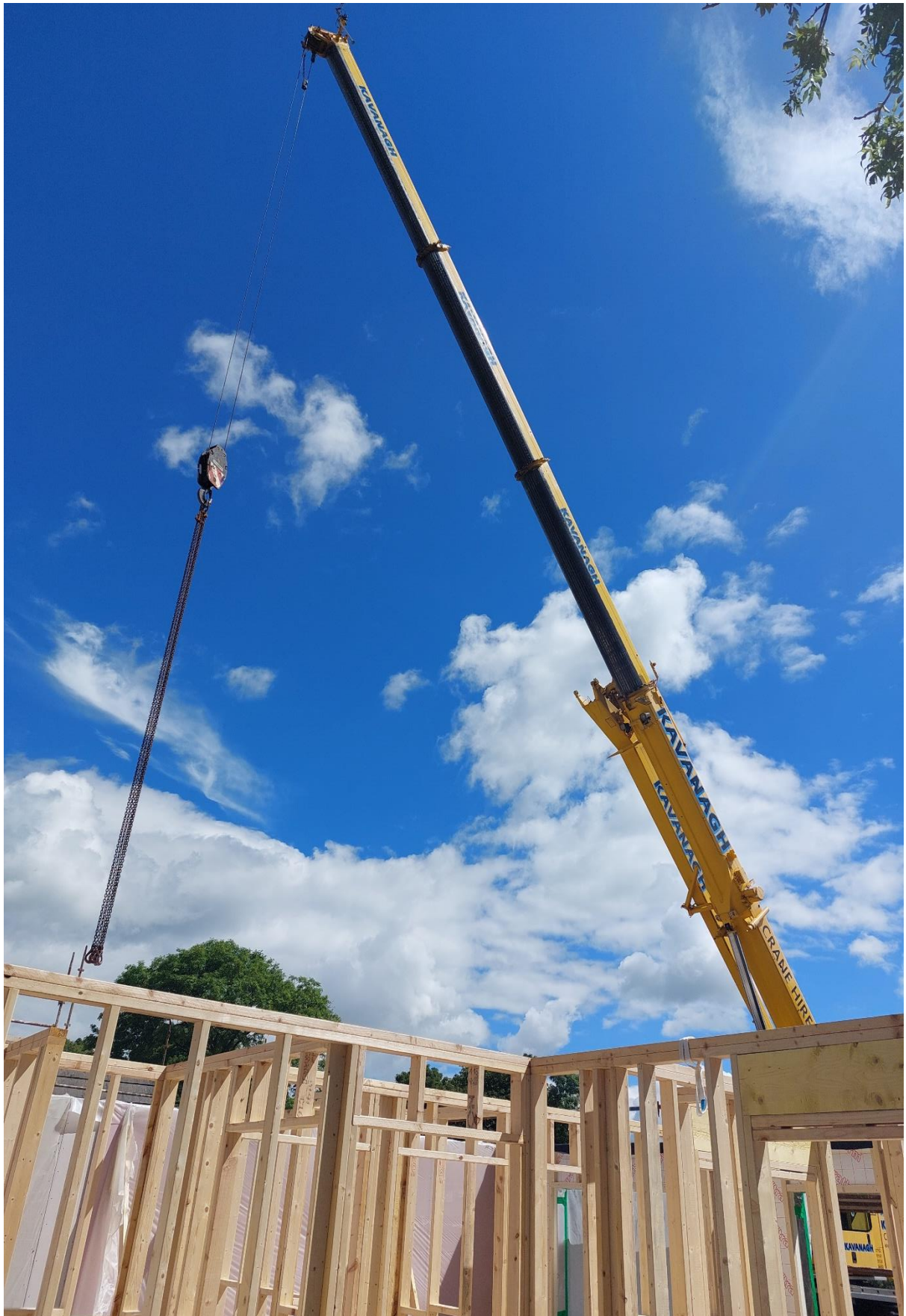
Erection of timber frame at Inchacarron Mullinavat. Low Carbon Construction.
