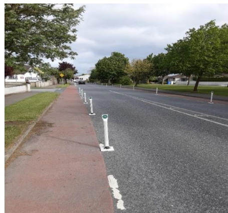
Provision of Cycle Bollards on Bohernatounish Road
