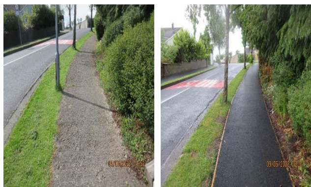
Footpath Repairs At Glendine Before & After
