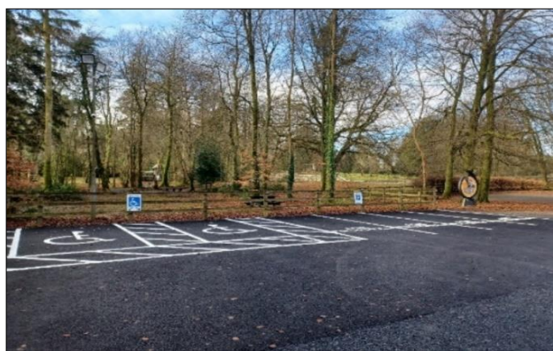
Recently installed Age Friendly & Disabled Parking Bays
