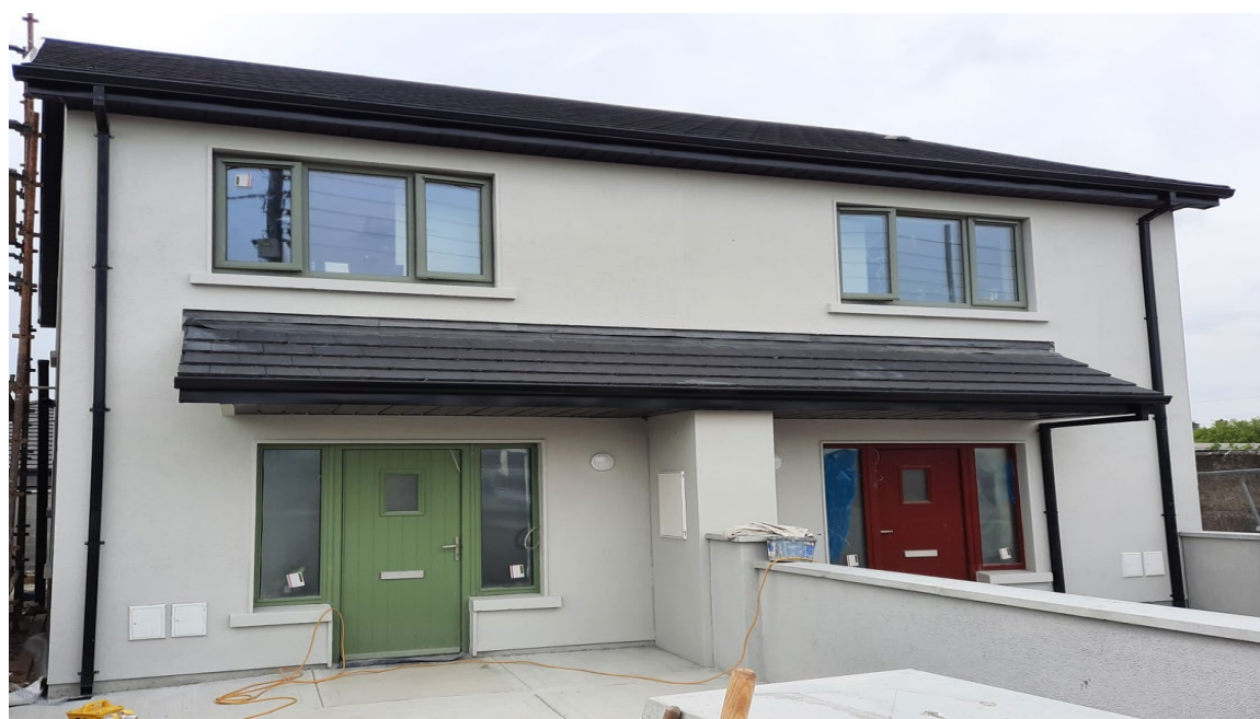
The above photos are of a bespoke disabled unit at Circular Road, Kilkenny which was allocated this month
