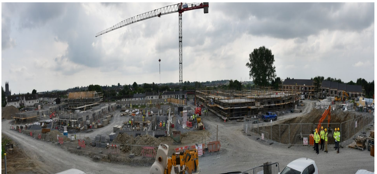
Construction Continues at Pace in Crokers Hill (photos above)
