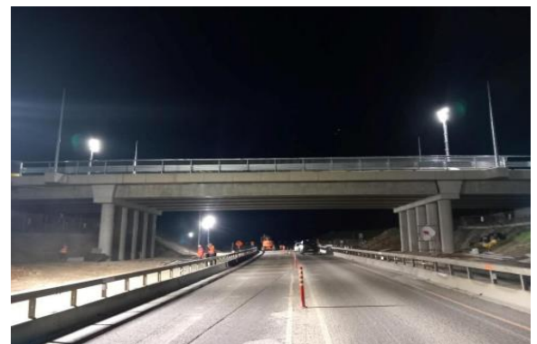
Nightworks on Bridge Structure
