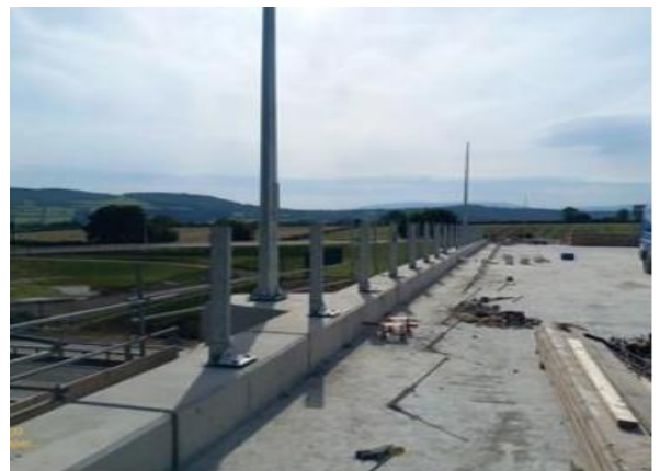
Bridge Parapet & Public Lighting Installation
