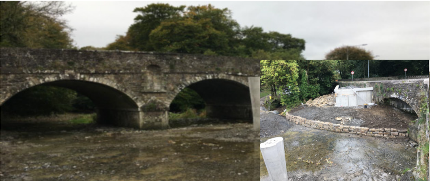
Central Pier Completed and river reinstated
