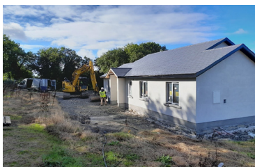
Construction of rural houses at Shanganny, Jenkinstown
