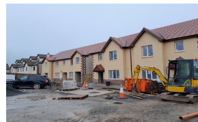
Construction at Limegrove, Belmont. 3 bed houses.
