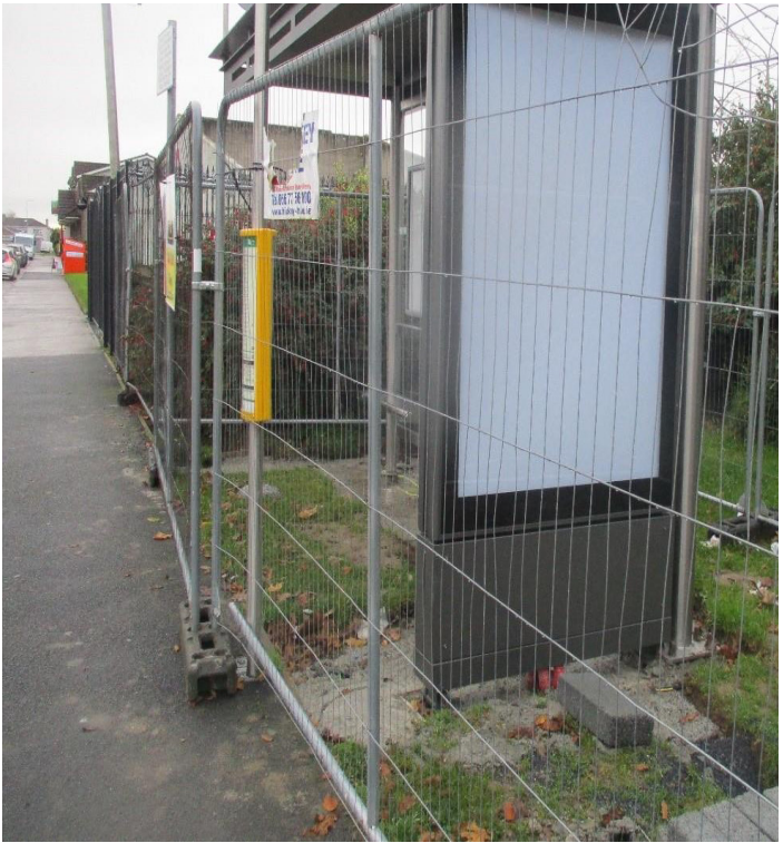
Bus Shelter Provision at Larchfield - SHELTER INSTALLED
