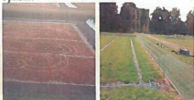
Setting out the topiary panels in the Winter Garden and the sunken panels with drainage and newly shaped terrace slopes
