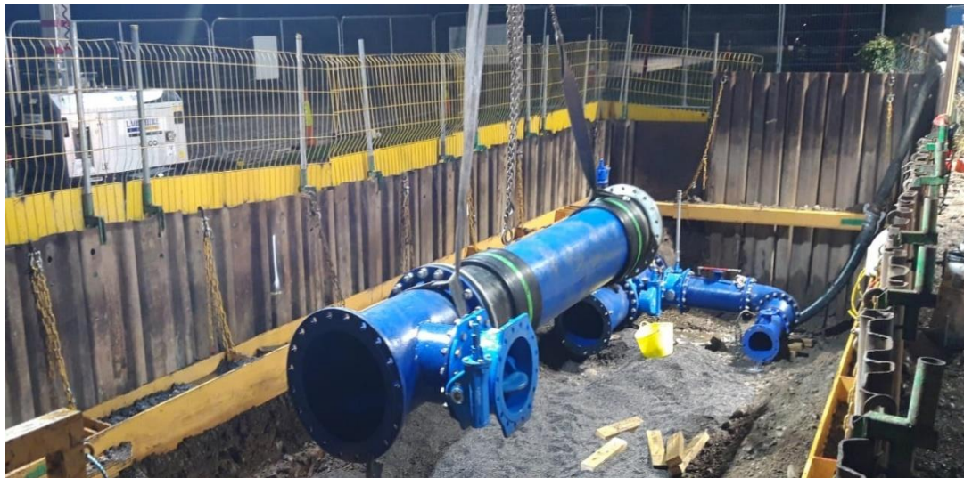
Installation of PRV in Kilkenny City February 2021
